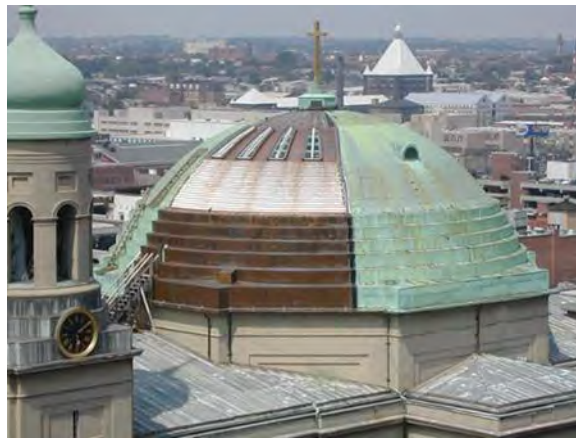
Figure 31 The twenty-four skylights in the dome were uncovered and new windows were installed. The original copper and wood shingle dome sheathing
