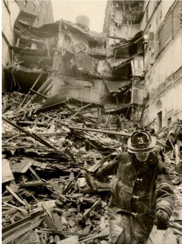
Figure 1.1 The Broadway Central Hotel on the day it collapsed in 1973, Michael Pollak, “Broadway Central Hotel’s Heyday Before a Fatal Collapse,” New York Times , Nov. 6, 2015. https://www.nytimes.com/2015/11/08/nyregion/broadway-central-hotels-heyday-before-a-fatal-collapse.html
