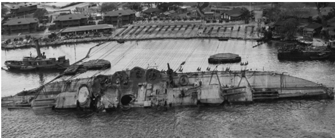
Taken on March 29, 1943, this image shows the USS Oklahoma (BB-37) righted back to about 30 degrees. Over a 6-week period, winches anchored on Ford Island slowly brought the ship back to a vertical position. Four months later the Oklahoma was fully refloated and moved to drydock. (Image courtesy of the Naval History and Heritage Command). 60
