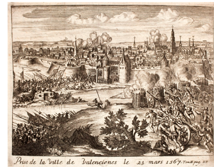
Figure 4: Siege of Valenciennes, 1567. Typical of the monetary constraints faced by many early modern states, the city of Valenciennes responded to artillery advancements by attempting to convert their medieval-era fortifications (rounded towers and thin curtain walls) to something which could withstand a modern siege. They shortened their walls and towers, backed them with earthen ramparts, and endeavored to mount artillery atop them. (From Strada, Famiano: De Bello Belgico Decades Duae (reprint 1727). Wikimedia Commons, Public Domain Image)
