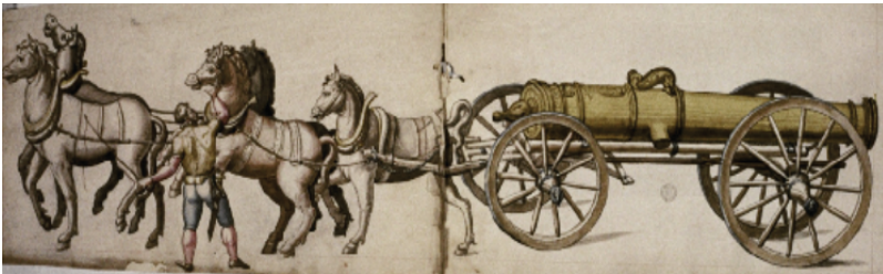
Figure 3: Advances in metallurgy and carriage construction, as well as gunpowder refinement, created the first truly mobile siege artillery. The power of heavy shot could, in a matter of days, raze walls which had withstood sieges of months and years in the previous era. (Dated 1582. Machines et ustensils de guerre ., whole page, Folio #: fol. 057r. Manuscript. Place: Bodleian Library, University of Oxford, http://www.bodleian.ox.ac.uk/ . https://library.artstor.org/asset/BODLEIAN_10310371924 .)
