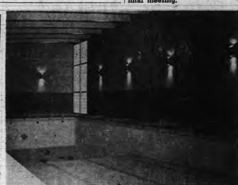
FINISHING TOUCHES did not come until late November, when plate glass and sound-proofing were added, and the spacious pool was tiled. Over-all length of the building is 215 feet, and the width, 183 feet.
