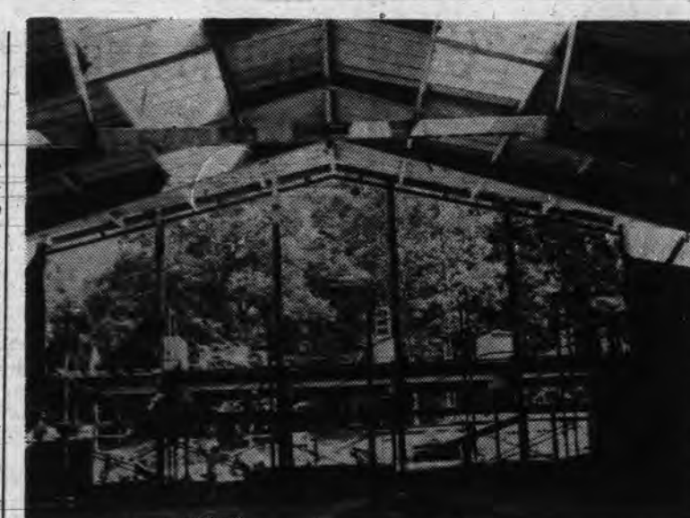
AS THE SUMMER PROGRESSED, construction showed rapid progress. Huge laminated arches were added, giving support to the brick and cinder-block walls which painters had splashed with modern blue, red, and green colors.
