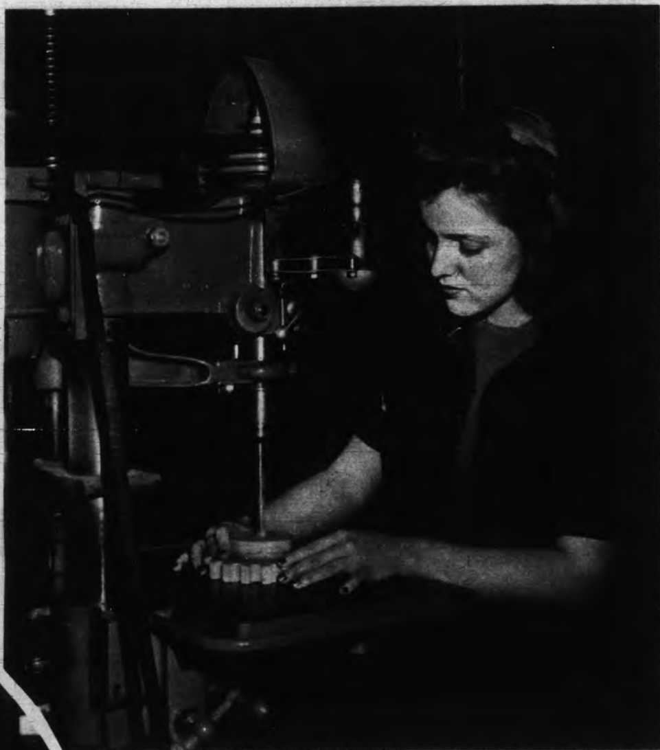
Wood Shop — Edna Thoma finishes a gear segment on a drill press. This pattern will afterwards be used to make a mold in the foundry, from which castings will be sent to the machine shop.
