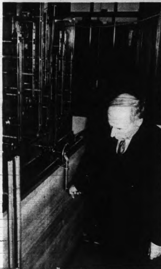
Does 61 Math Operations at Once Weighing a ton and looking almost like a creation from Mars, this multihermograph invented by Dr. S. LeR. Brown, University of Texas, is the only instrument in the world that can solve equations up to the fifteenth degree.
